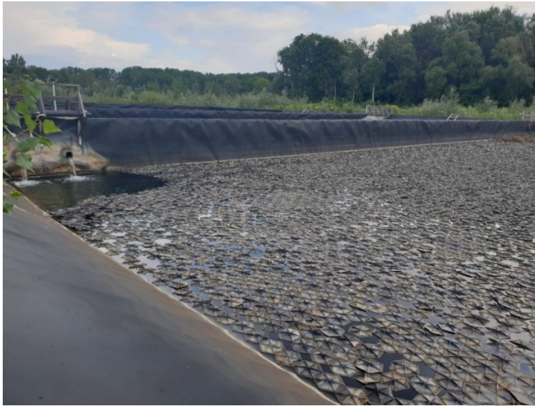
Figure 6: Basin C – before the start of the sTES planning process (Planungsgruppe M+M AG, 2013).
