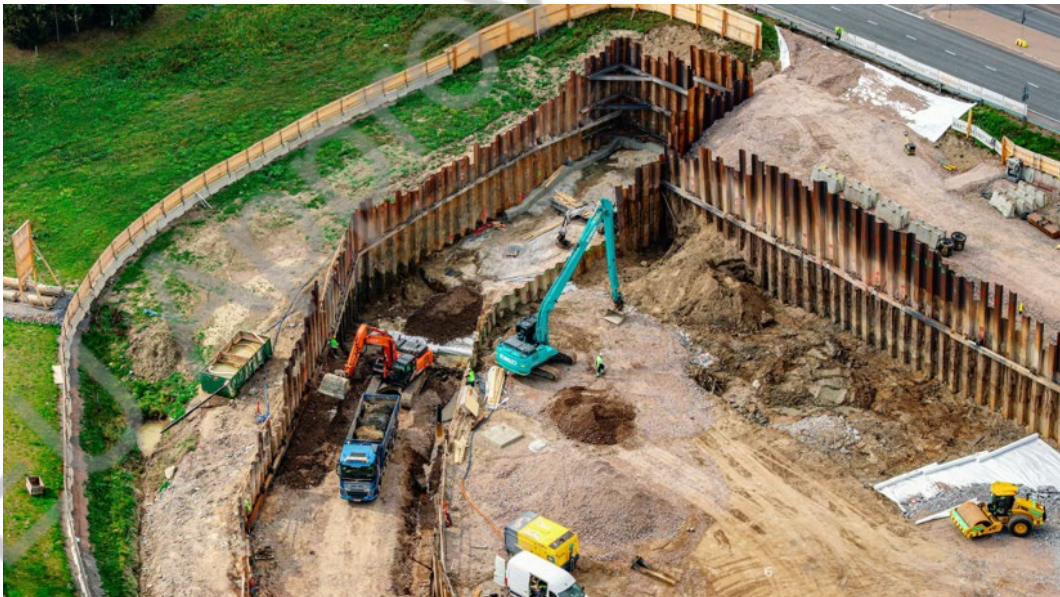
Figure 58: A closer view of the construction at the service entrance.
