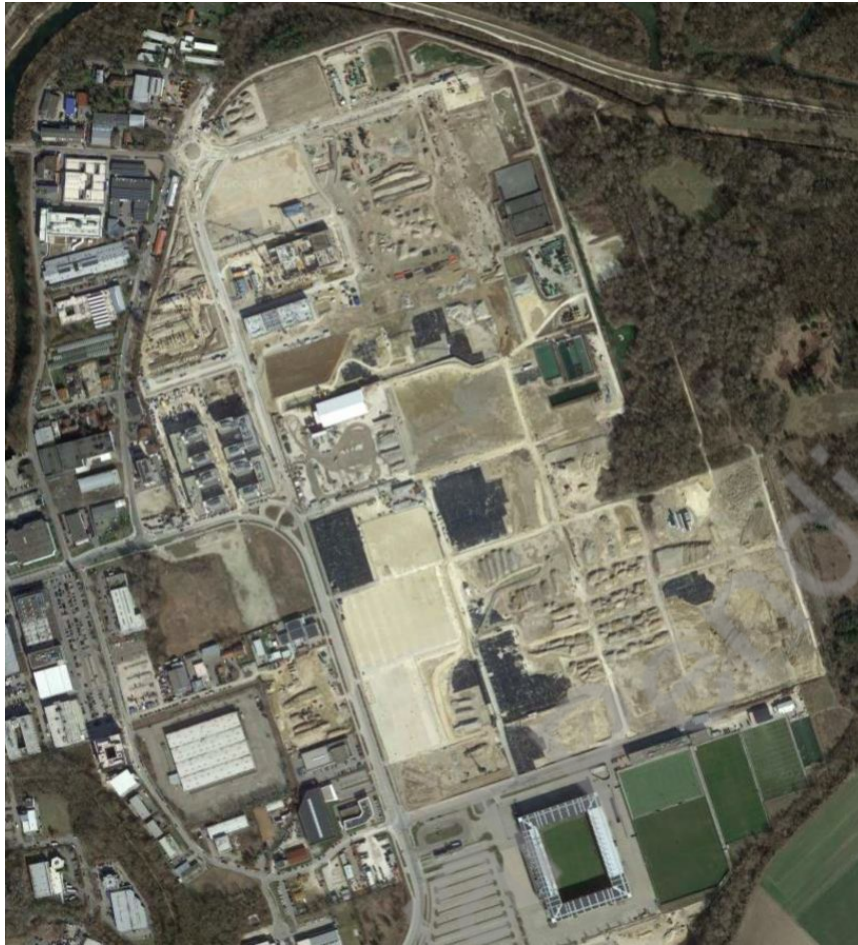
Figure 2: Demo site (Ingolstadt, Germany) after the dismantling in 2020 (Audi, 2024).
