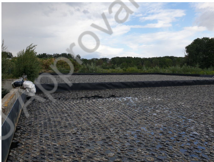
Figure 5: Basins A + B – before the start of the sTES planning process (Planungsgruppe M+M AG, 2013).
