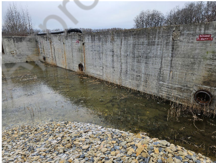
Figure 7: Pump station after the demolition (Planungsgruppe M+M AG, 2013).
