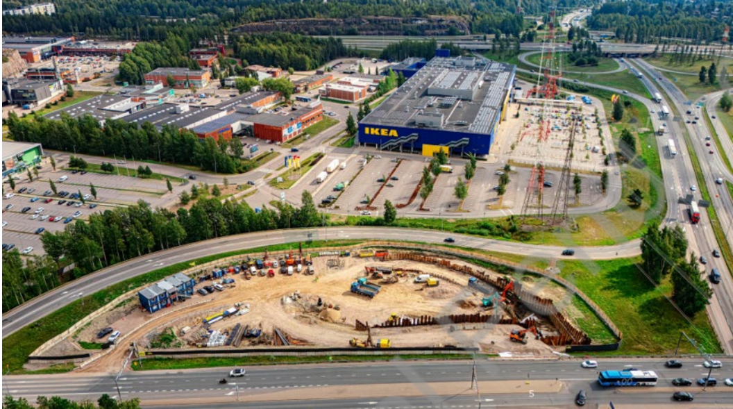
Figure 57: Above-ground construction work at the service entrance for the Varanto storage.
